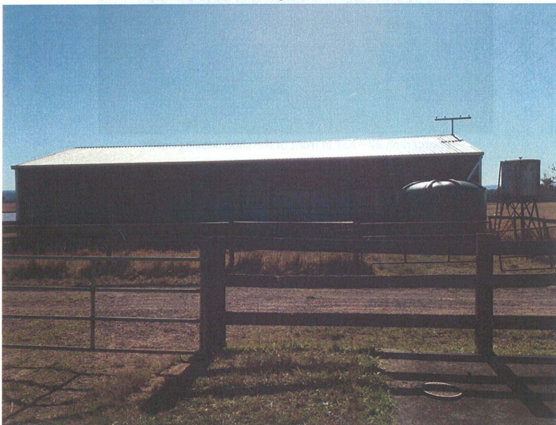
Photograph 26 – Shed behind the residential complex, looking north west.
