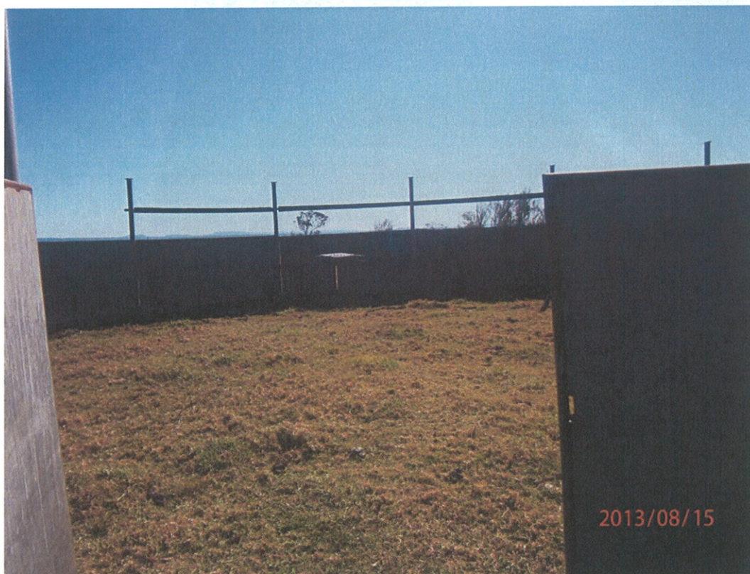
Photograph 17 – Wooden structure in northeastern portion of lot 201, facing northwest.
