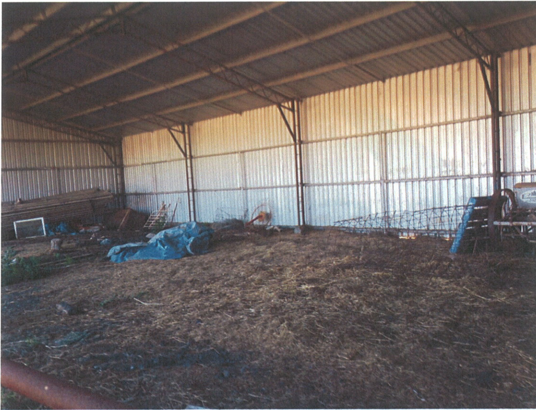
Photograph 28 – Material stored within the shed.
