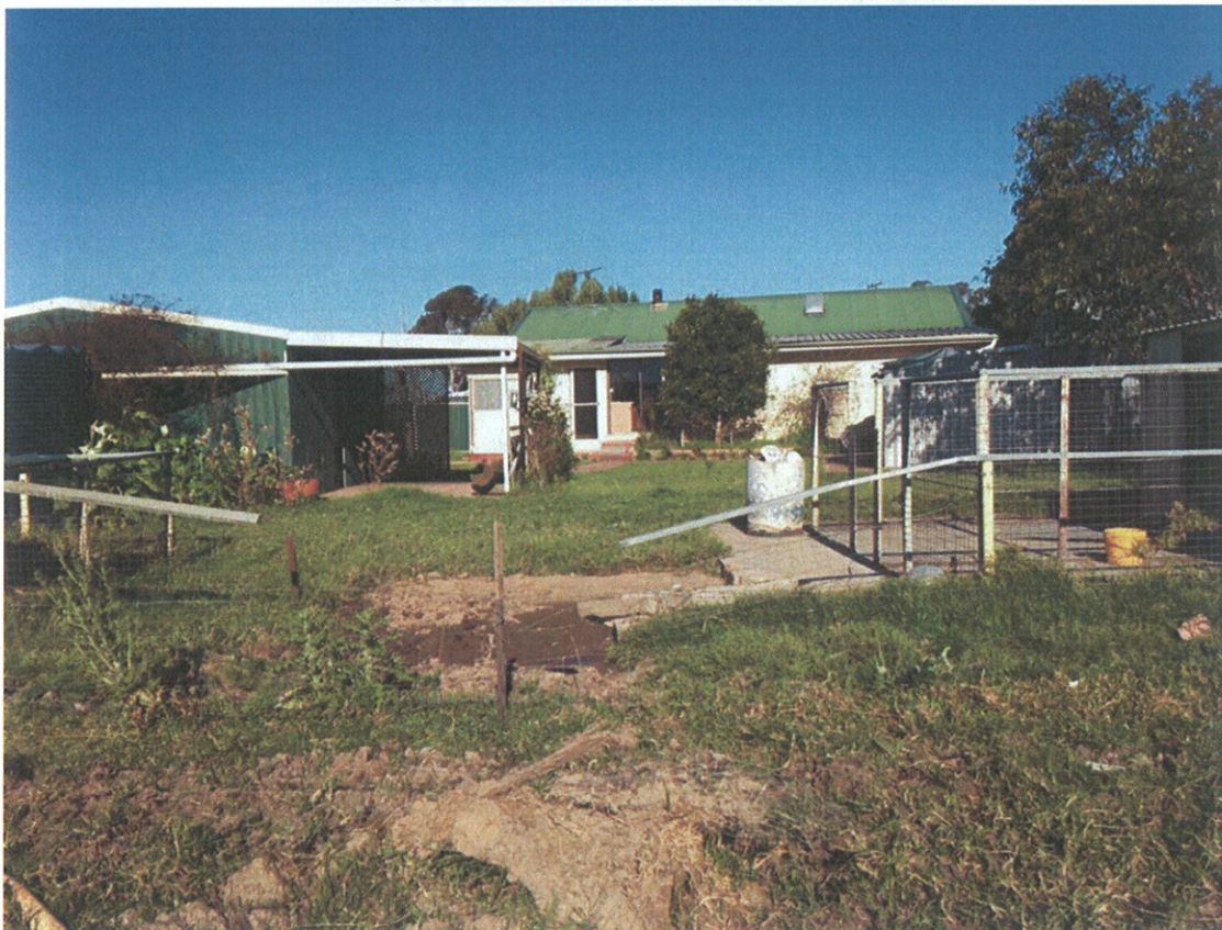
Photograph 43 – Rear of residence 3, looking southeast.
