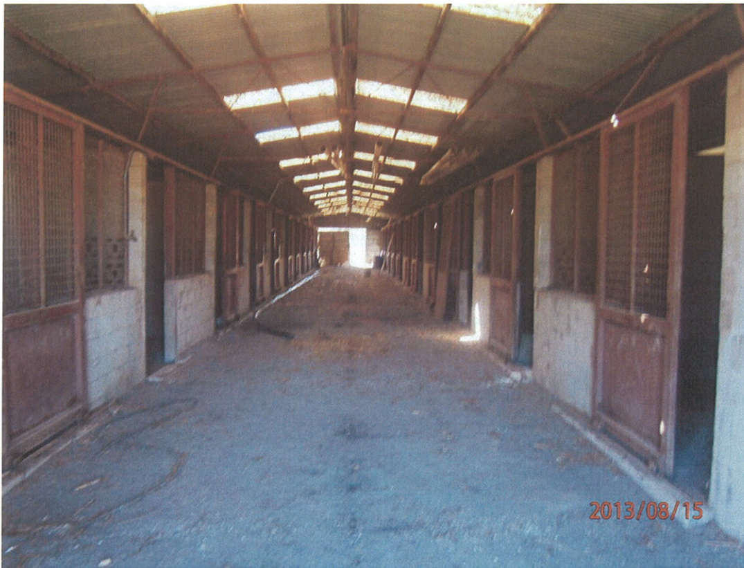
Photograph 15 – Stable shed in the northeastern portion of Lot 201
