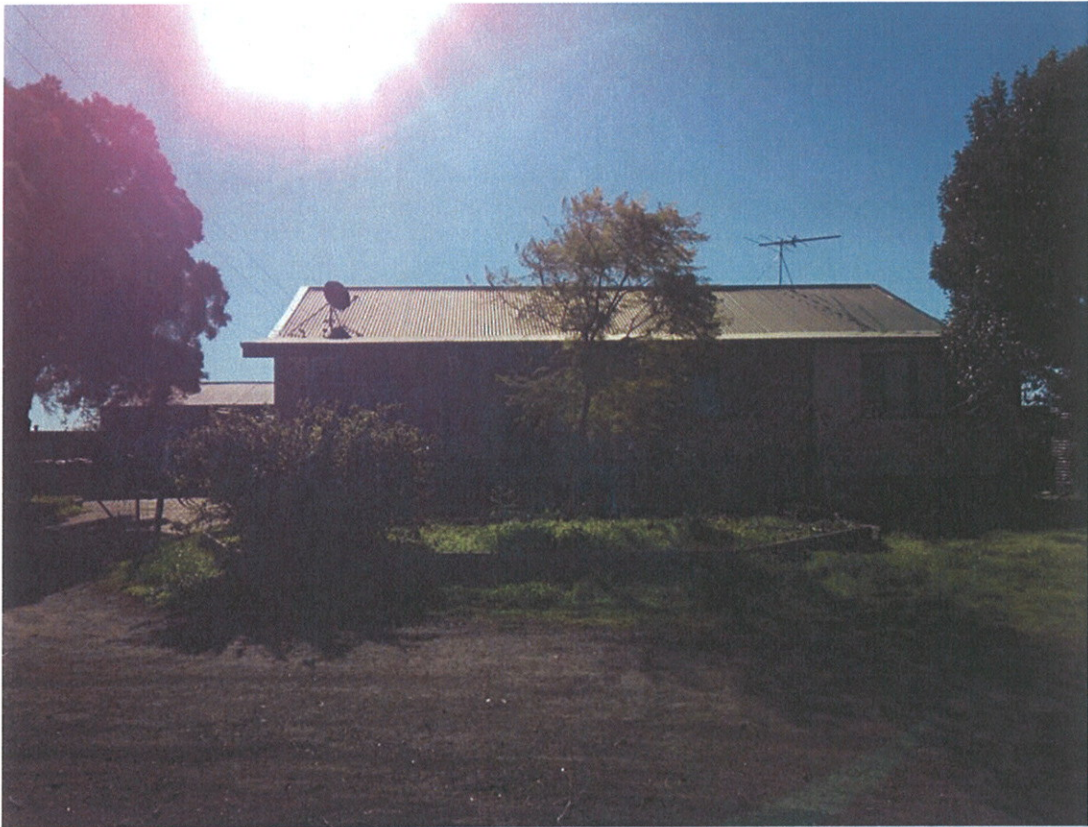
Photograph 42 – Residence 3, looking northwest.
