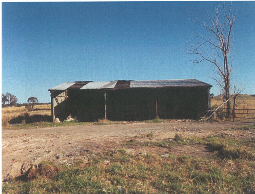
Photograph 47 – Shed southwest of residence 3 looking south.
