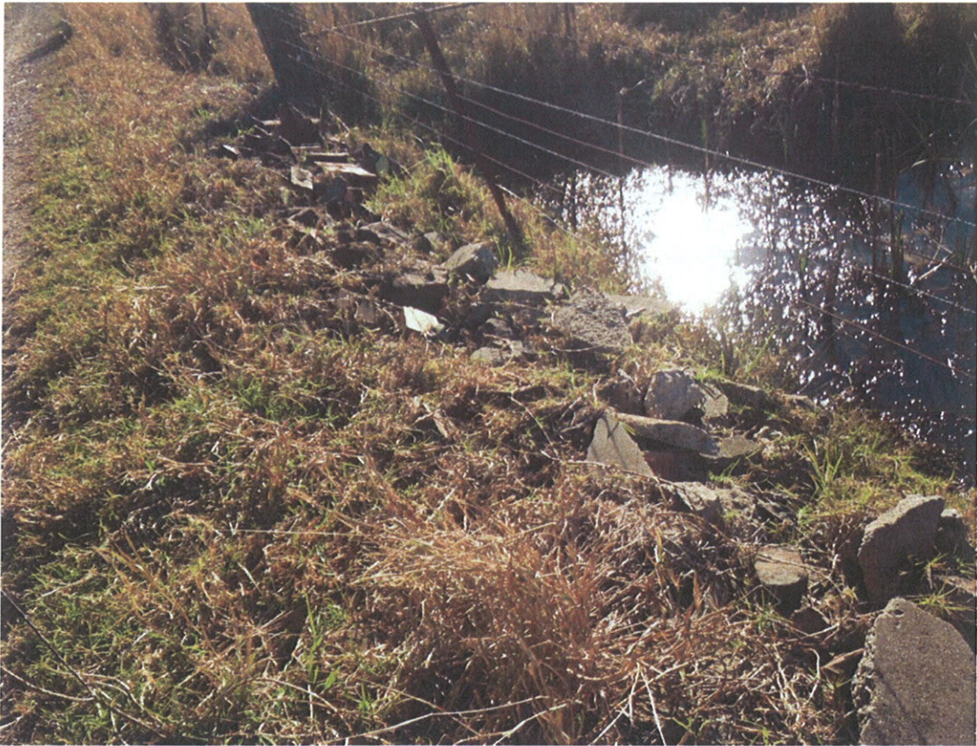
Photograph 40 – Fill material in the main access road of the site.
