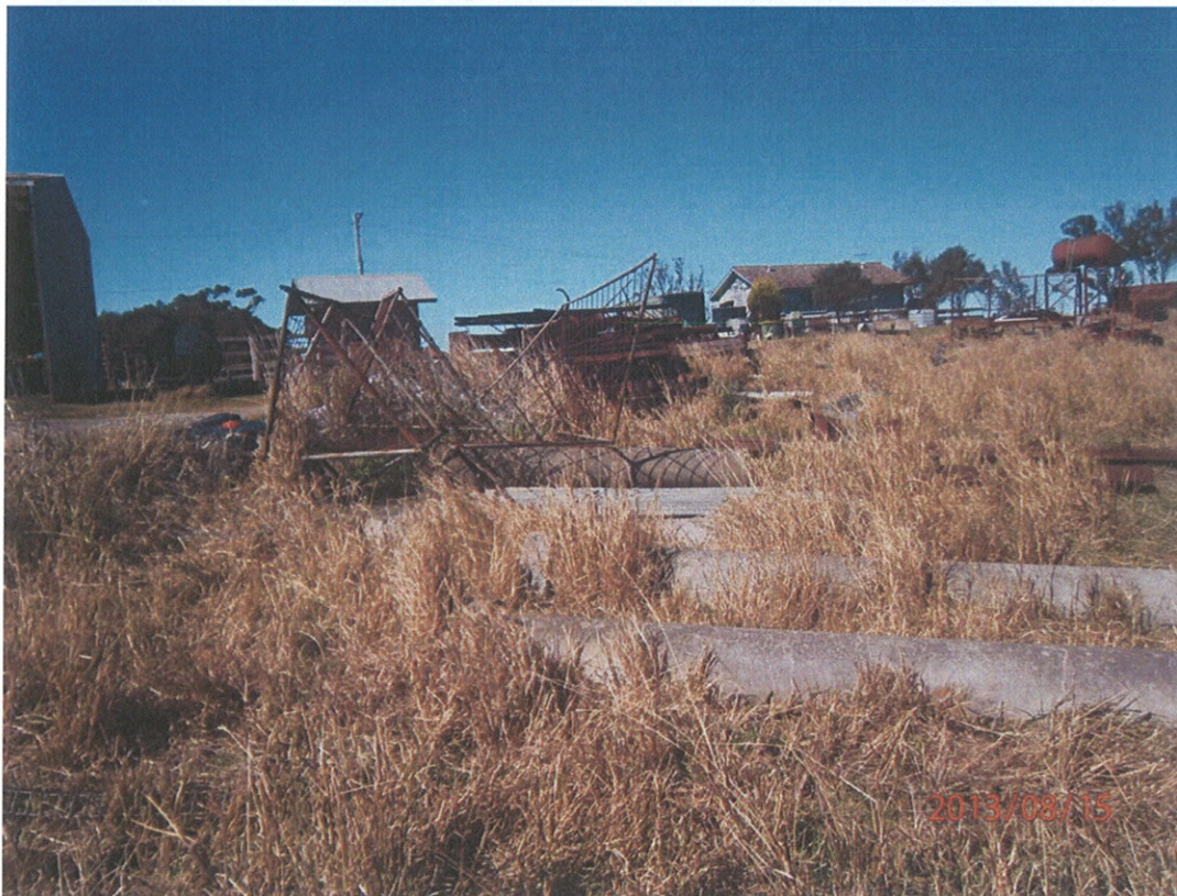
Photograph 20 – Suspected ACM pipe and steel stockpiles west of the house in the southeastern portion Lot 201, looking east.
