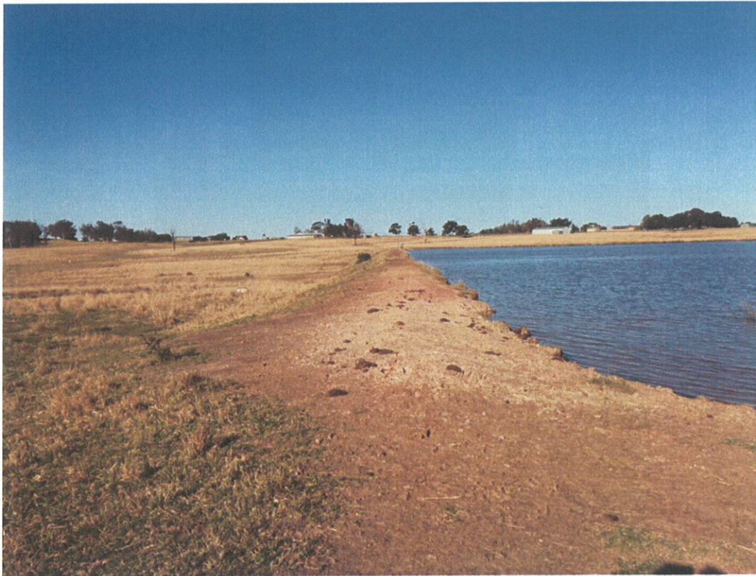
Photograph 32 – Northern dam wall of the large dam in the Western portion of Lot 201, looking east.
