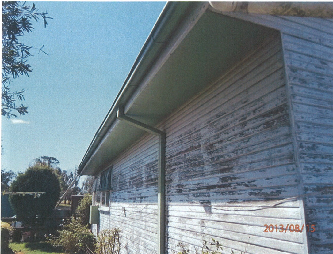
Photograph 11 – ACM eaves of north eastern house.
