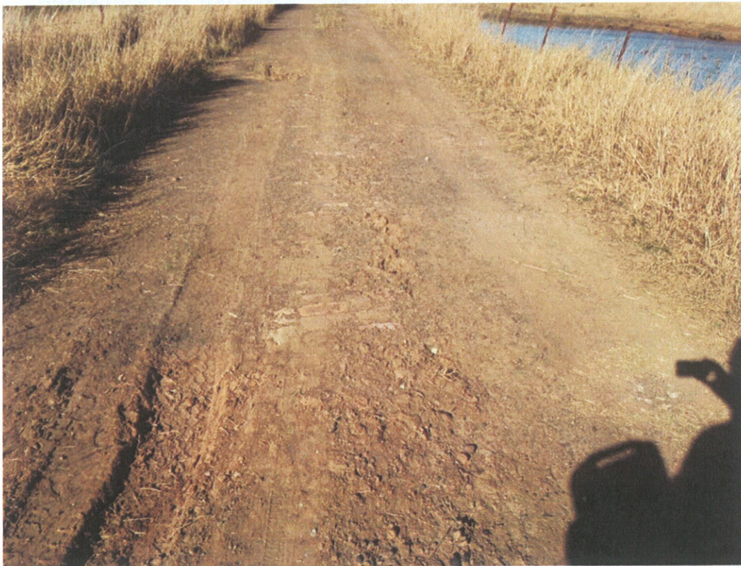
Photograph 39 – Fill material in the main access road of the site.
