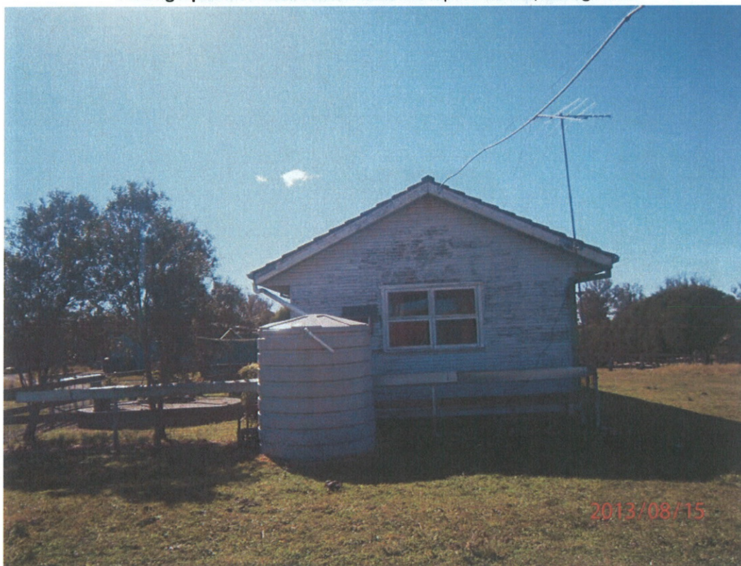
Photograph 10 – The rear of the house (Residence 1) in the northeast of Lot 201, facing north.
