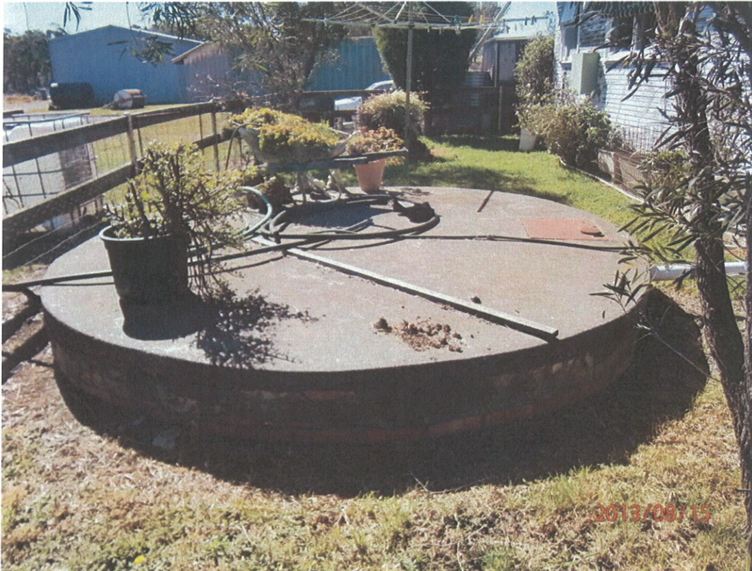
Photograph 13 – Septic tank west of the northeastern house
